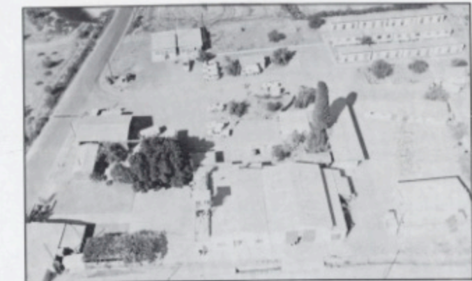
Aerial view of Camp Izay
