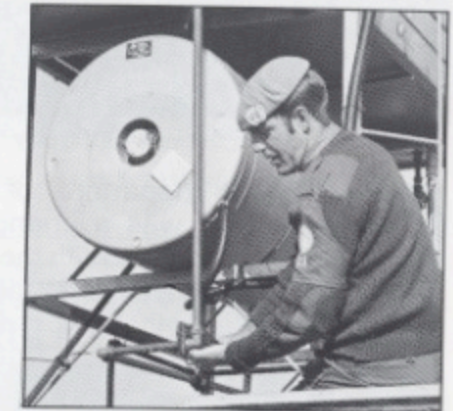
Cpl Morph Moreby plumbing in a hot water system
