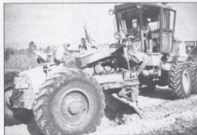
LCpl Murphy shaping the track to the correct crossfall
