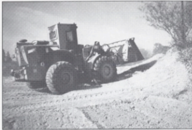
Equipment for airfield damage repair being used in friendlier situations
