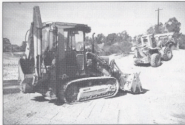
Equipment used during the demolition of the YMCA underground bunker
