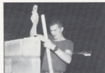
LCpl Diston showing his skills in bricklaying
