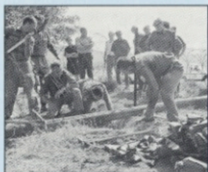
The FC gets an overview of an underground problem
