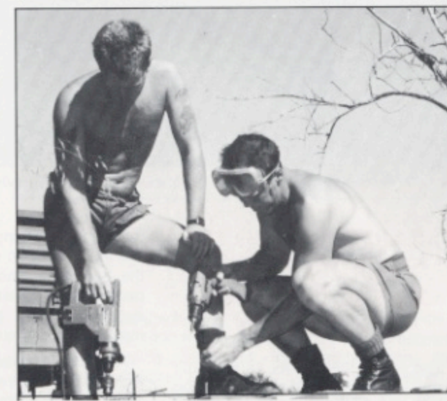
Cpl Parker assisting LCpl Woodcock in laying decking for bridge
