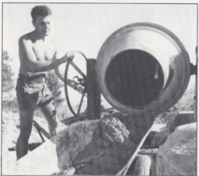
2Lt Piers-Vickers mixing cement for abutment facing
