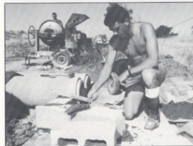
Spr Martin laying blocks for the culvert supporting walls
