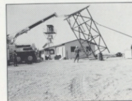
Erecting a new tower for the sentry box
