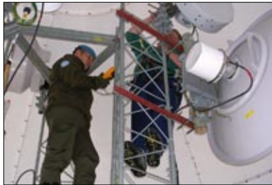
Installing microwave links in the dome
