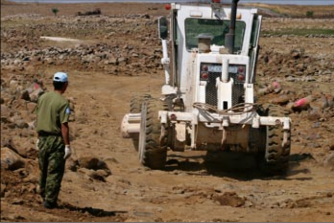
Level the ground with a grader
