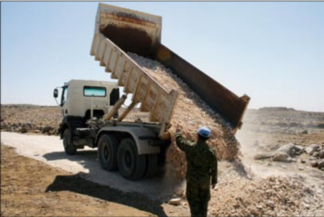
Unload gravel for road construction
