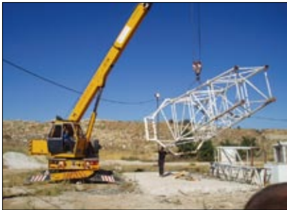
Build-up of a watch tower
