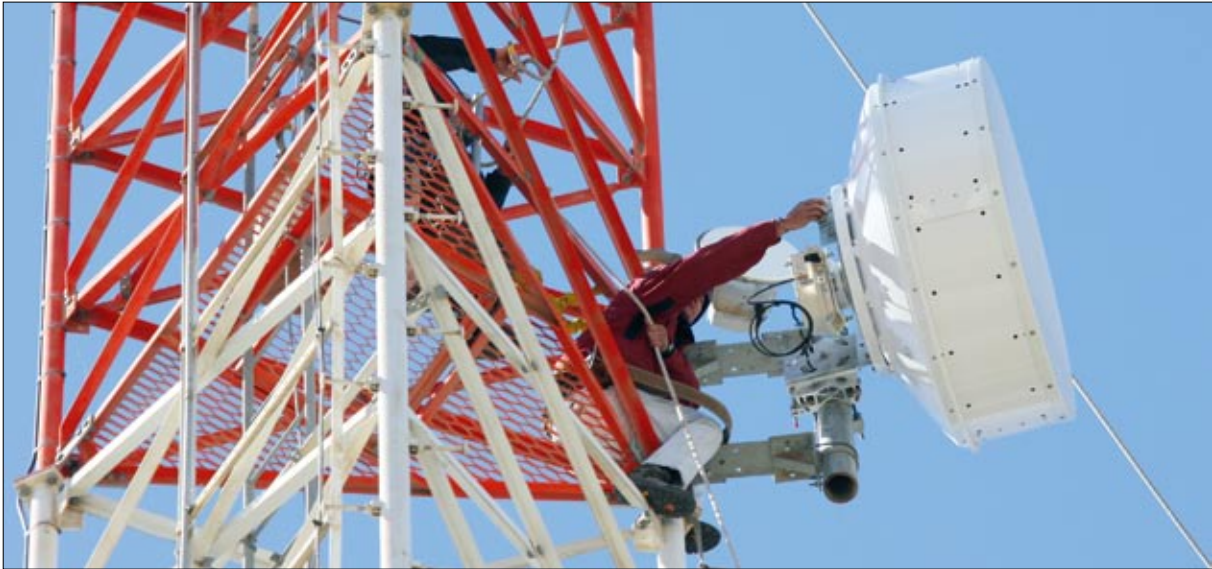
Alignment of the microwave link
