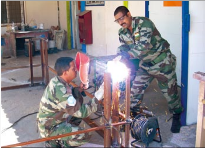
Engineers welding an iron frame
