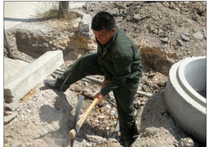
A signaller runs cables
